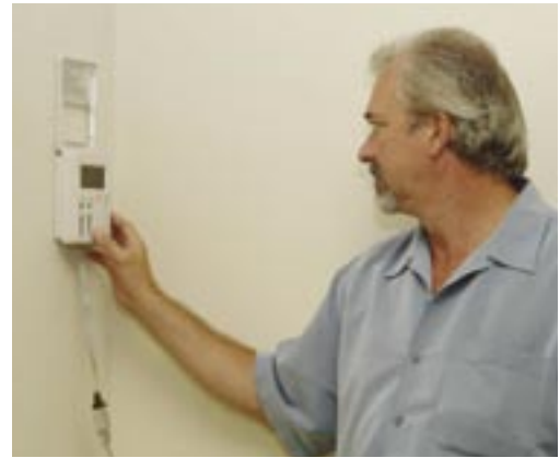
Mike Nelson of R-Cold, Inc. demonstrates how to adjust the settings on the Beacon II System using the Beacon II Smart Controller.
